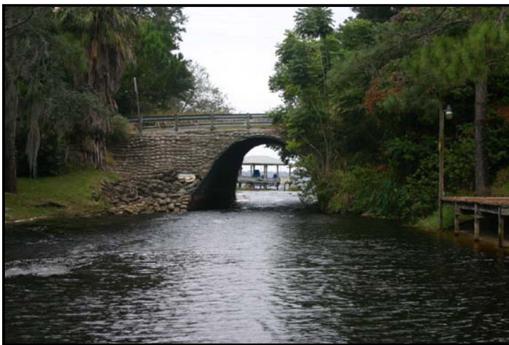
Figure 2. Montevista Canal Culvert between Crescent Lake and Lake Minnehaha.
