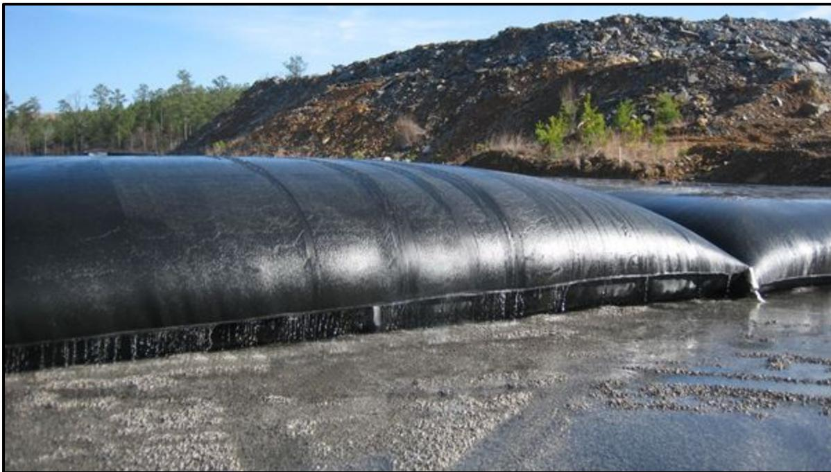
Figure 2. Photograph of large geotube like those proposed for the NuRF.
